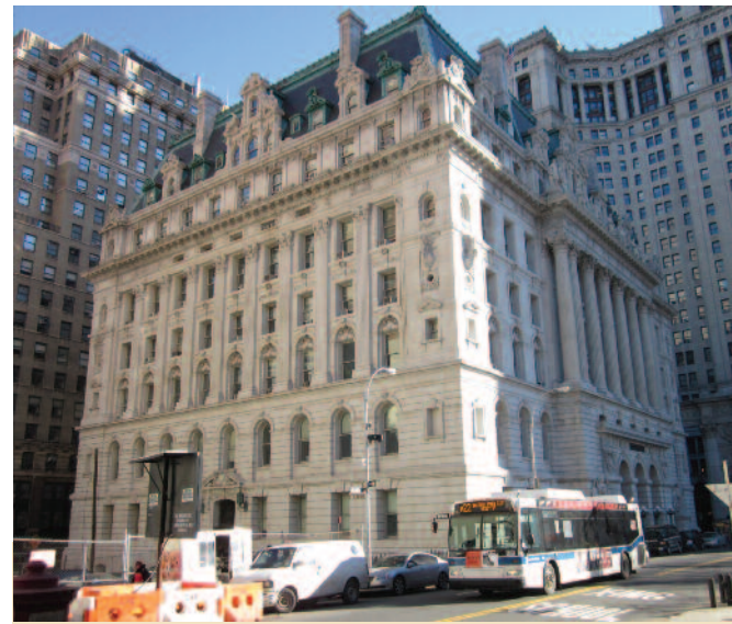
The New York City Public Administrator's Office, this year's Starnet Design Award "Unique Installation" category winner, was renovated throughout with low profile access flooring.
